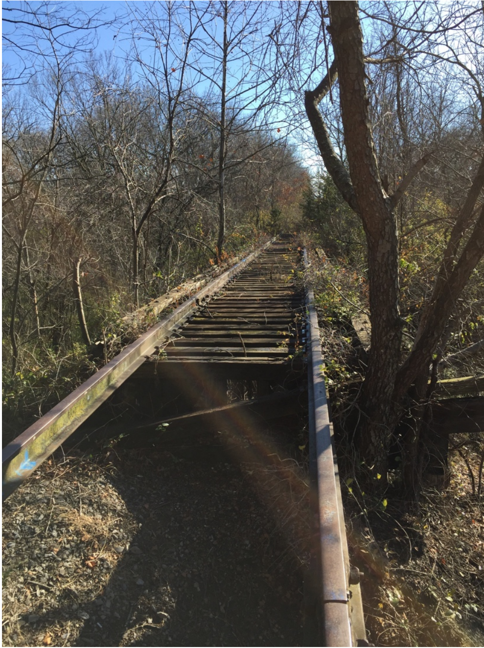
Bridge at MP 281.5. View from deck looking southeast. Date: December 5, 2016
