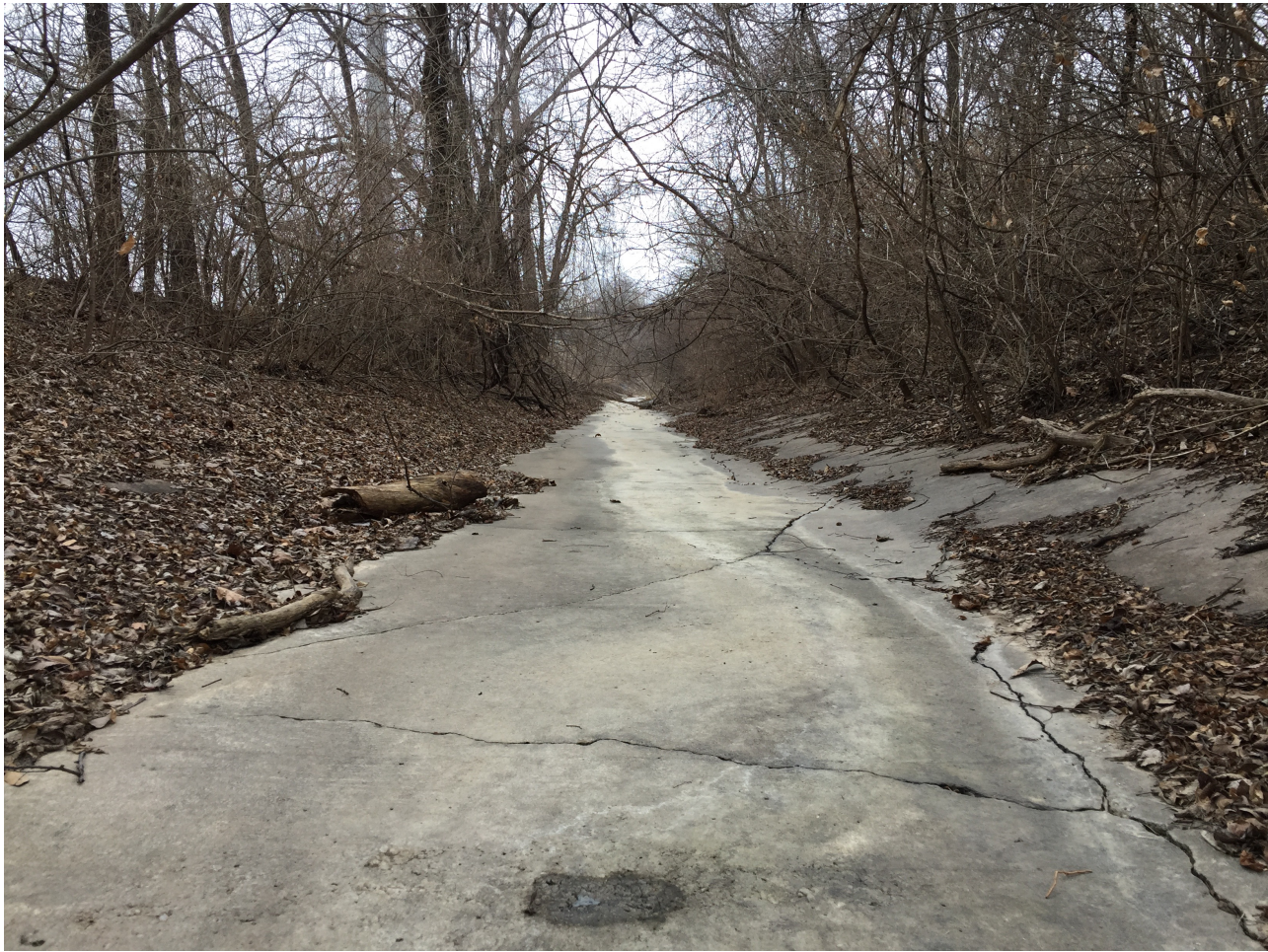
Weir at MP 286.2, Kansas City. General view facing south. Date: February 7, 2017
