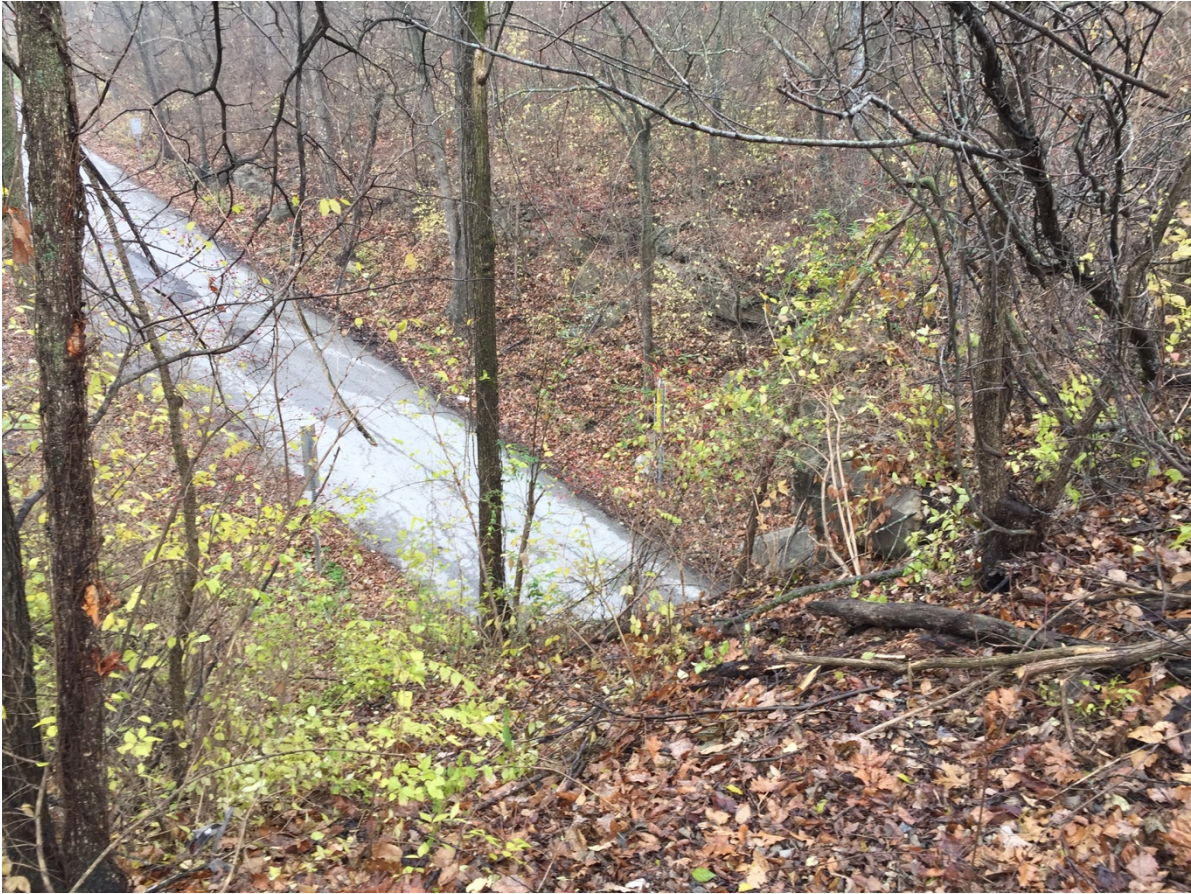
Bridge at MP No. 280.00 over Frost Road, Raytown, MO. View from the deck of the bridge toward Frost Road. Date: December 6, 2016
