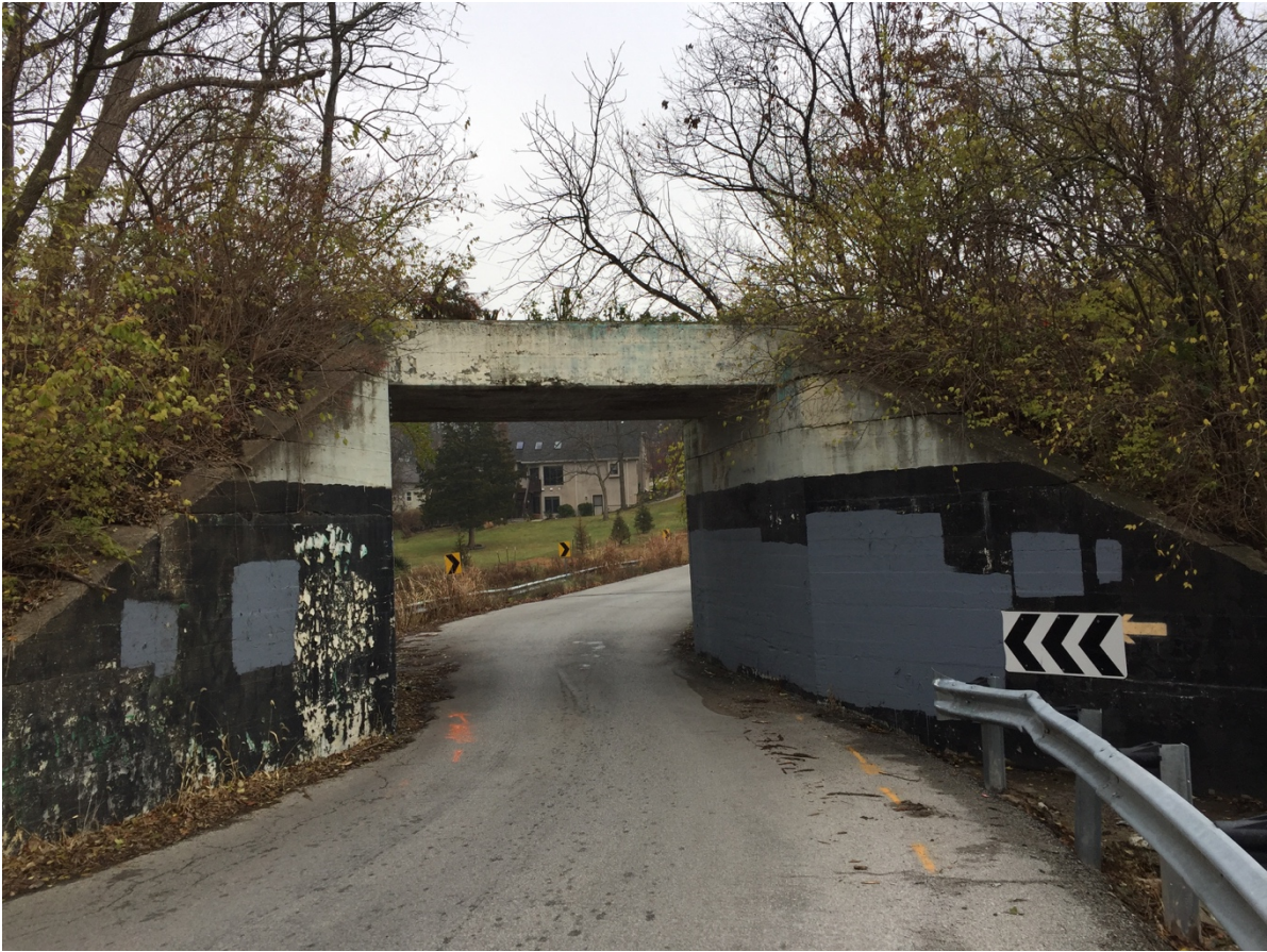
Bridge at MP 280.6. View of west façade, looking east. Date: December 5, 2016
