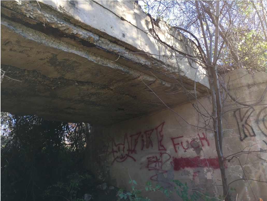
Bridge at MP 282.4, Raytown, MO. General view of the west façade looking east (above); detail of the abutment and I-beam encased in concrete looking southeast (below). Date: December 5, 2016.
