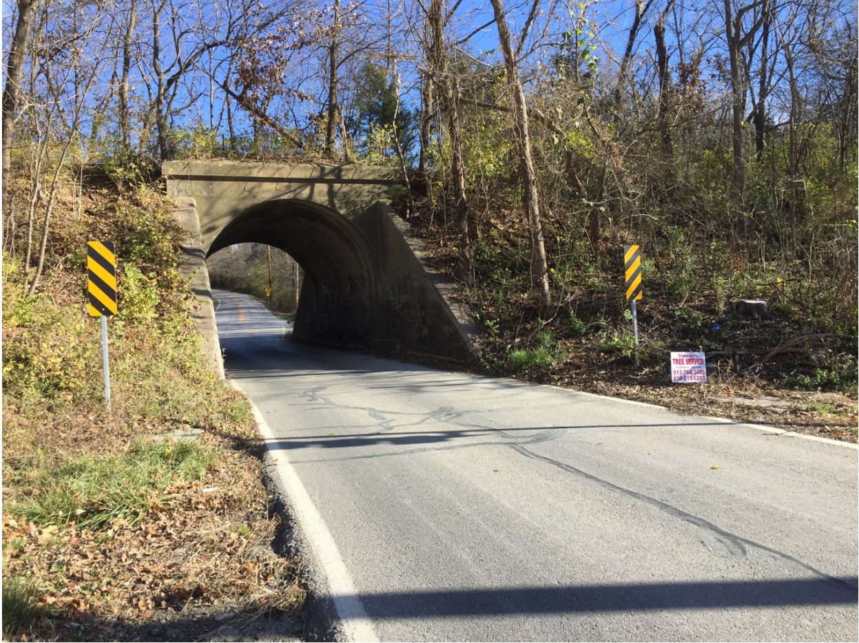
Bridge at MP 276.3, Chipman Road, Lee's Summit. View of west façade, looking east. Date: December 6, 2016
