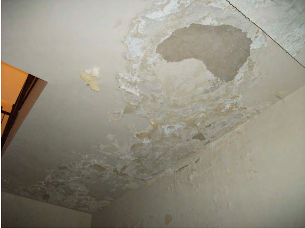
Second Floor East End Room 204
