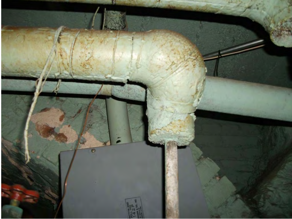
Homogenous Area M – Elbow on Cork Pipe Cover
