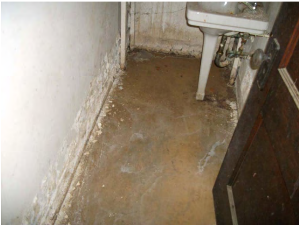
Basement East End Room 006
