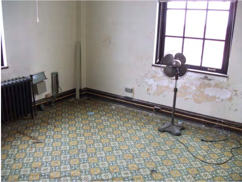
Second Floor West End Room 228
