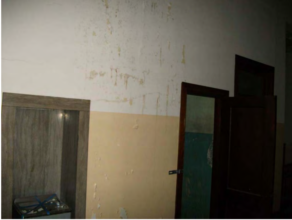
Second Floor West End Room 203
