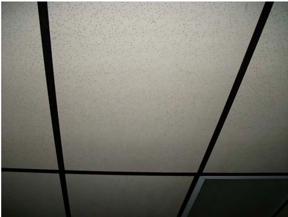
Homogenous Area BB – 2x4 Pinhole Pattern, Drop Ceiling Tile
