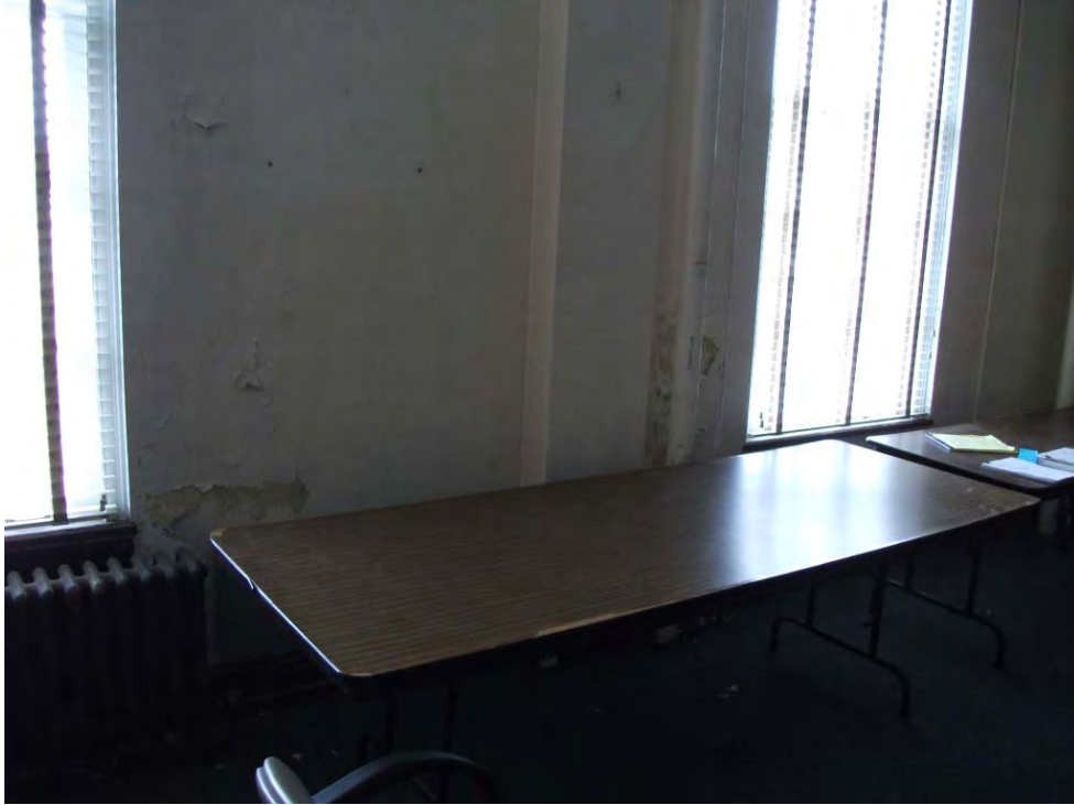
First Floor West End Room 144
