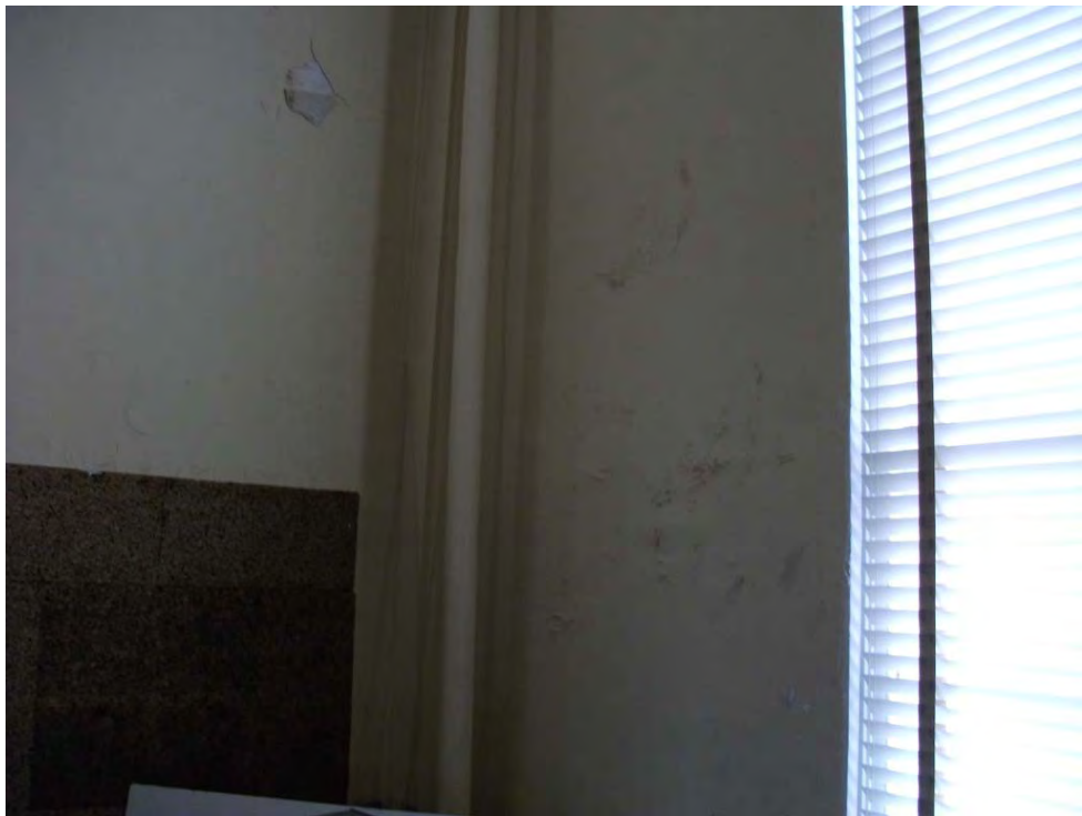
First Floor East End Room 133
