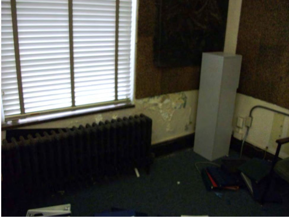
First Floor West End Room 139
