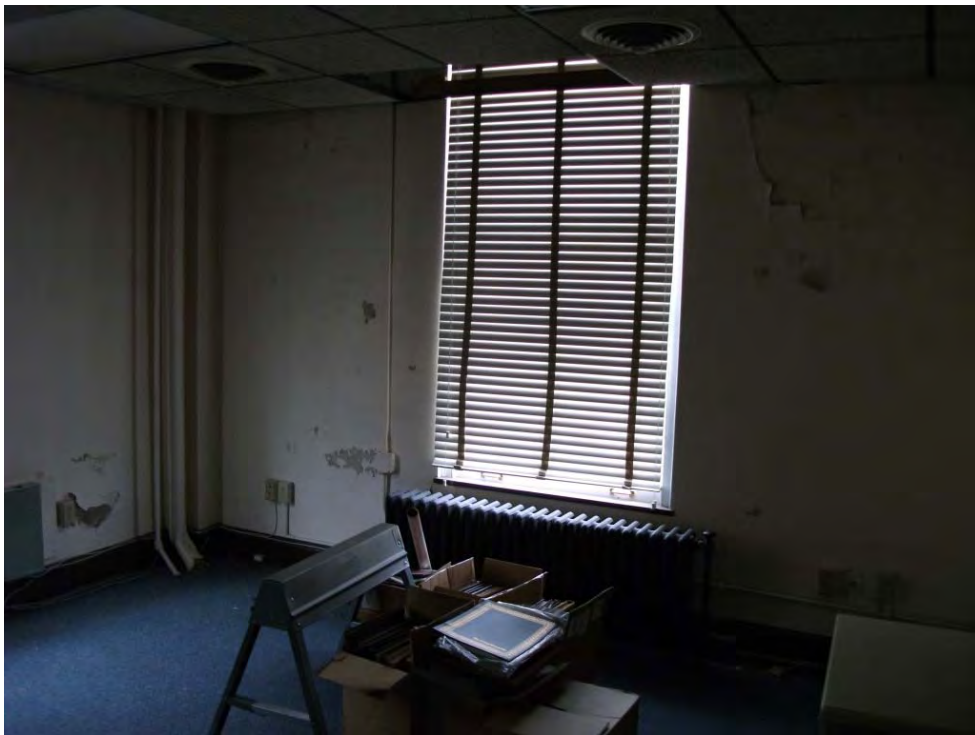
First Floor West End Room 145
