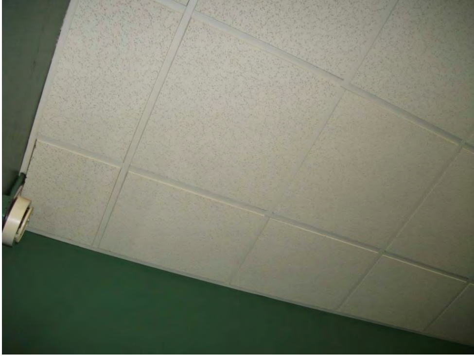
Homogenous Area O – 2x2 Worm Pattern, Drop Ceiling Tile
