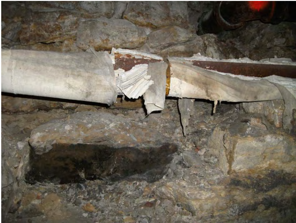
Homogenous Area H – Air Cell Pipe Cover
