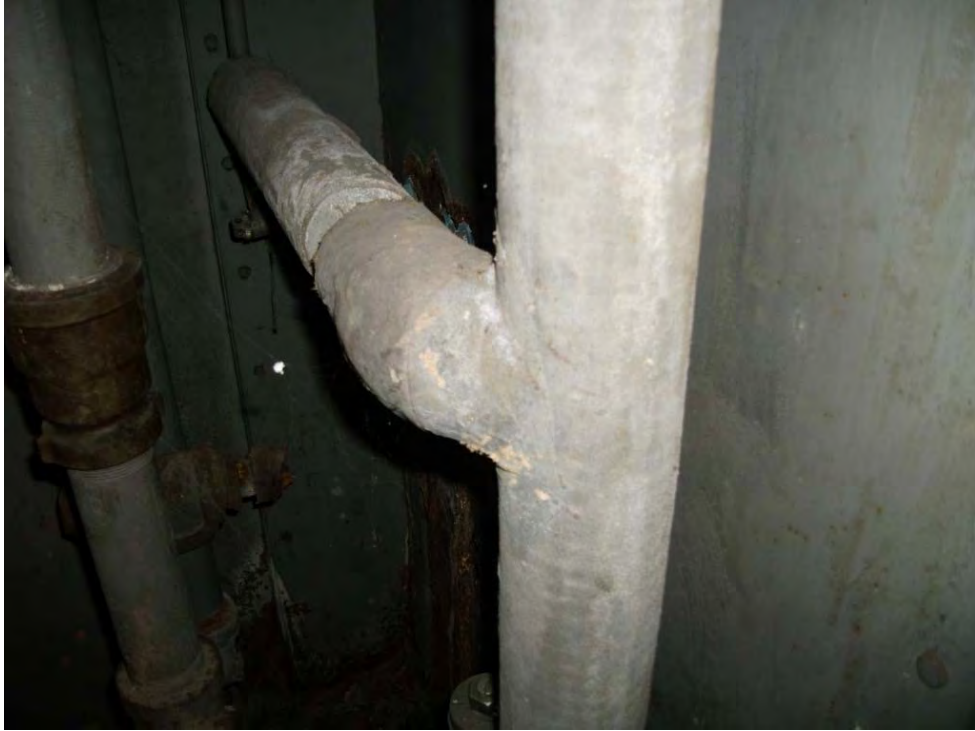
Homogenous Area K – Mudded Joint Packing on Wrapped Paper Pipe Cover
