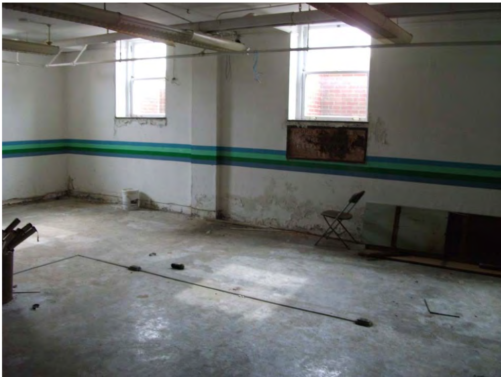
Basement East End Room 002
