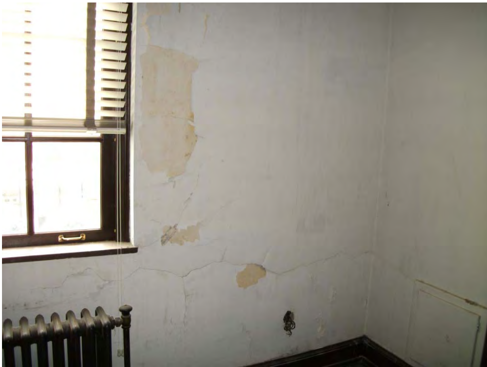
Second Floor East End Room 251
