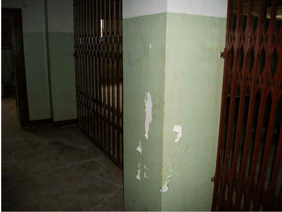
Basement East End Room 002
