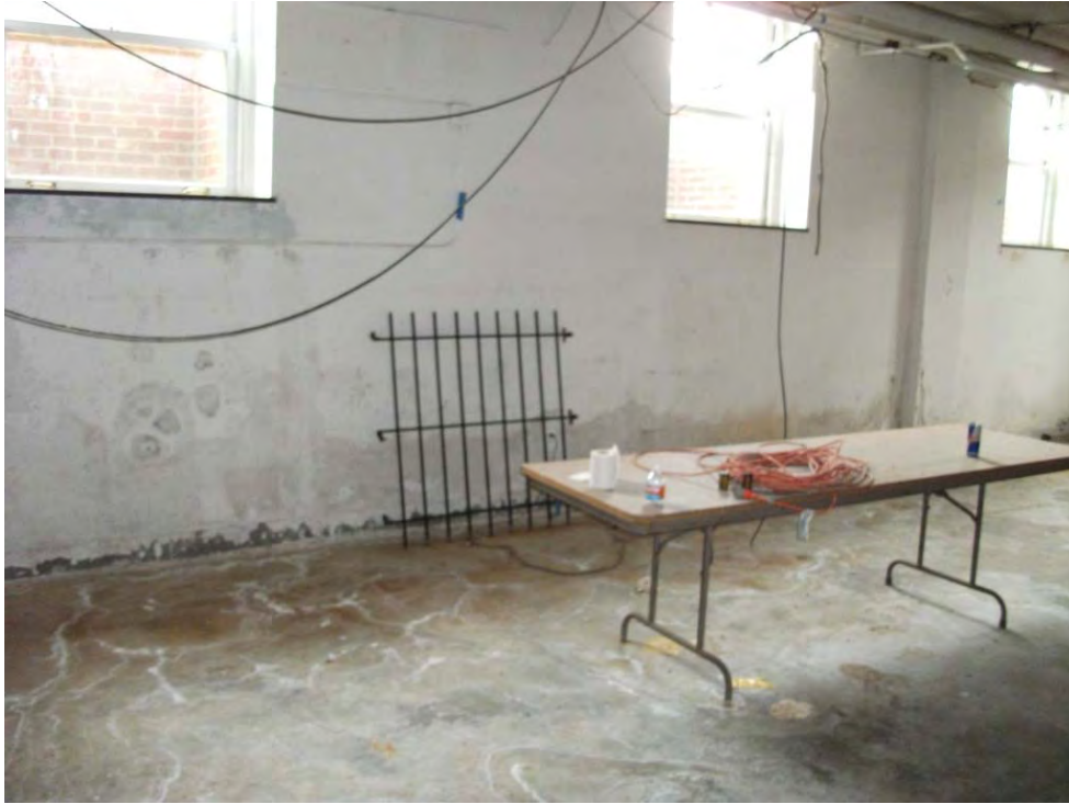
Basement East Side North End
