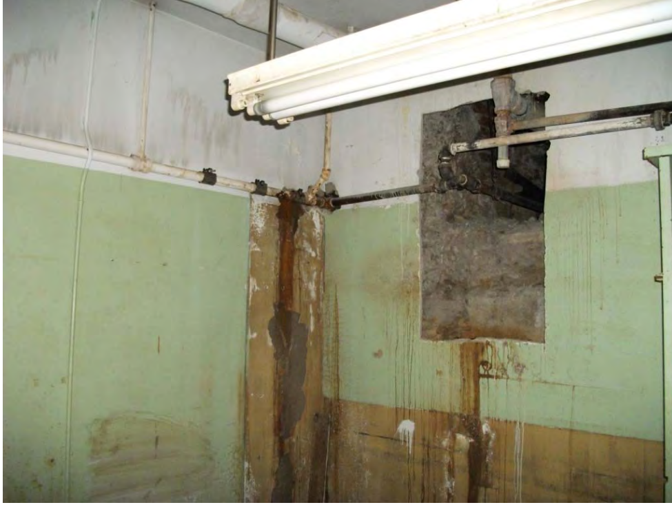
Basement East End Room 008
