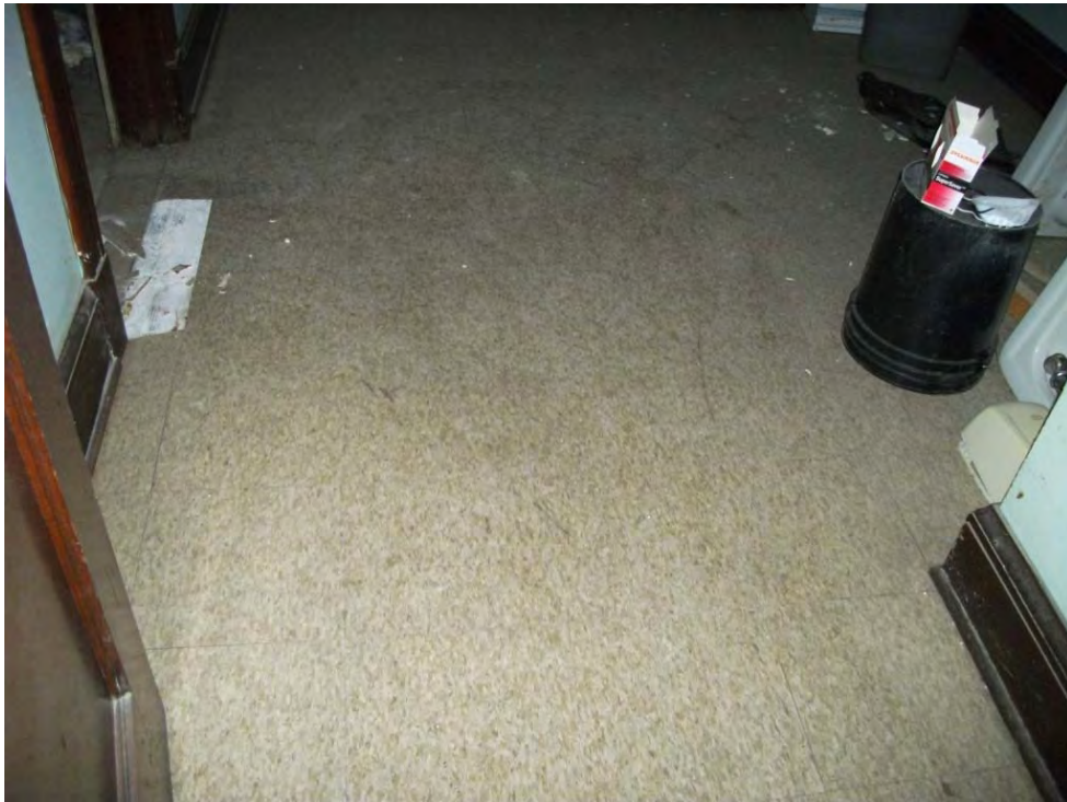
Homogenous Area D – 12x12 Brown Vinyl Floor Tile
