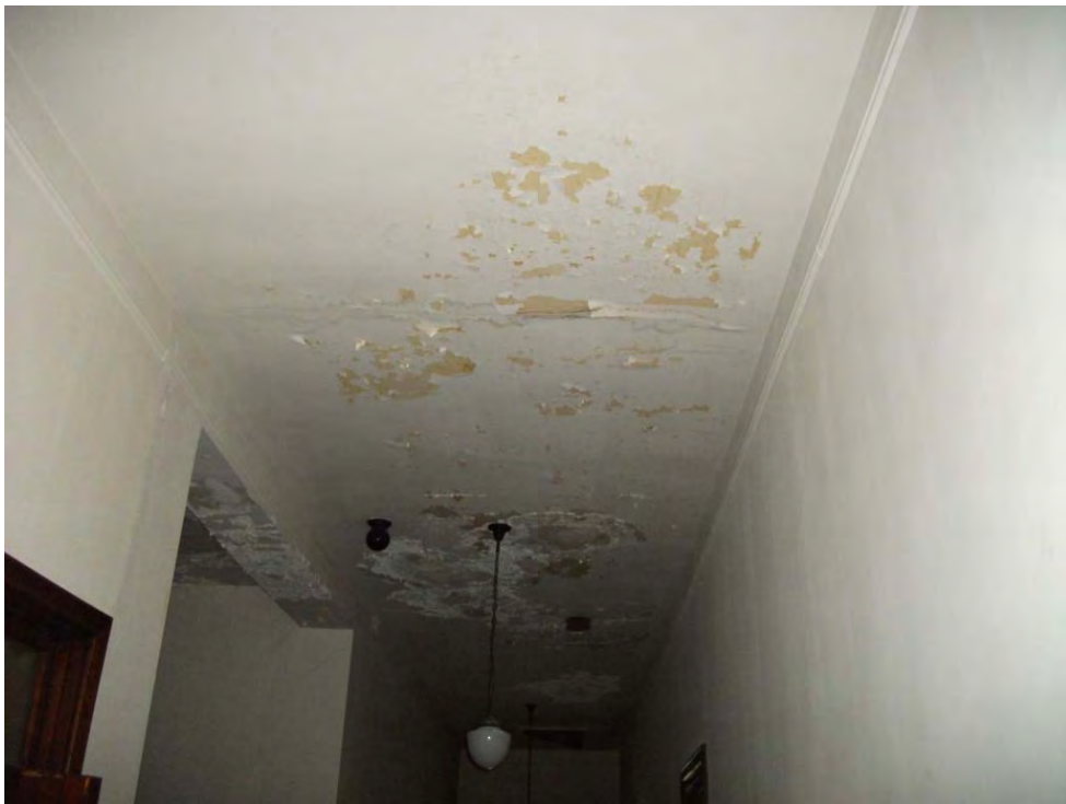
Second Floor East End Room 202
