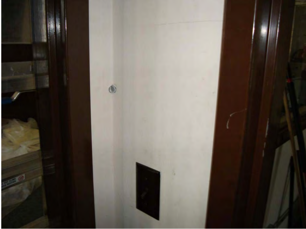
Homogenous Area Q – Drywall
