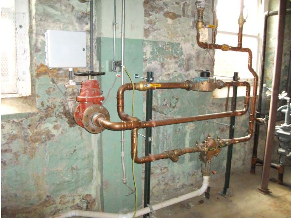
Basement West End Room 010
