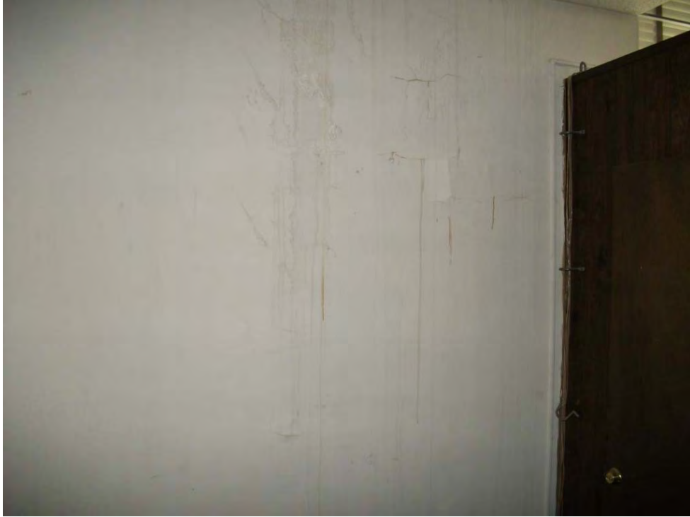
Second Floor East End Room 252
