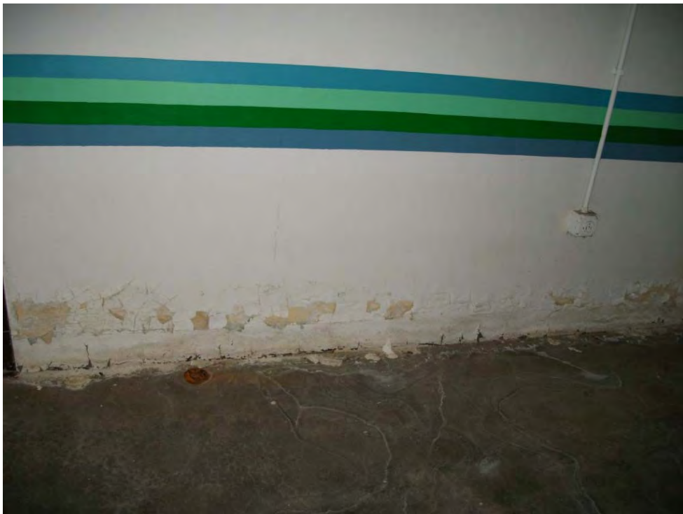
Basement East End Room 002
