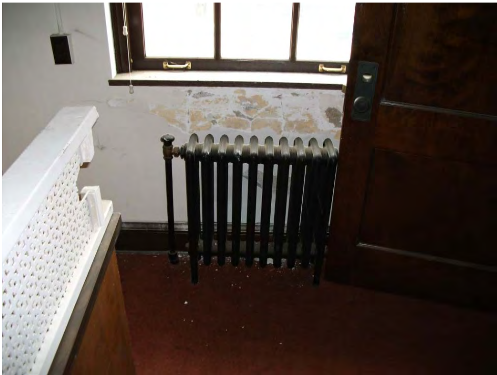
Second Floor East End Room 248
