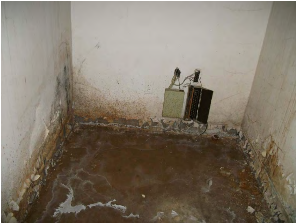
Basement East Side Room North of Vault
