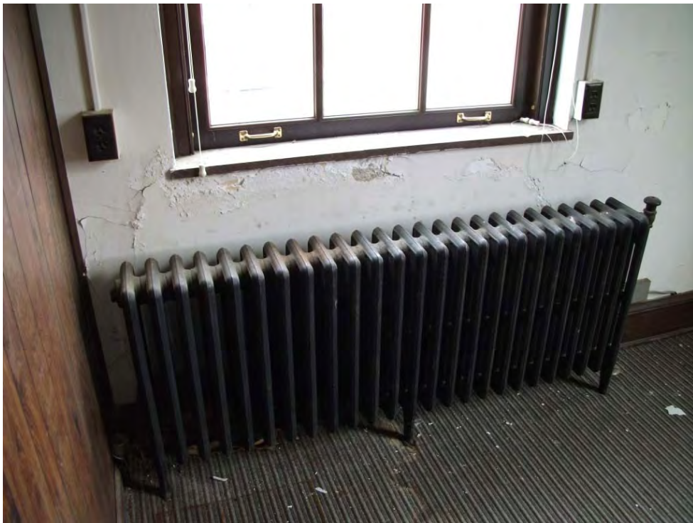
Second Floor East End Room 252
