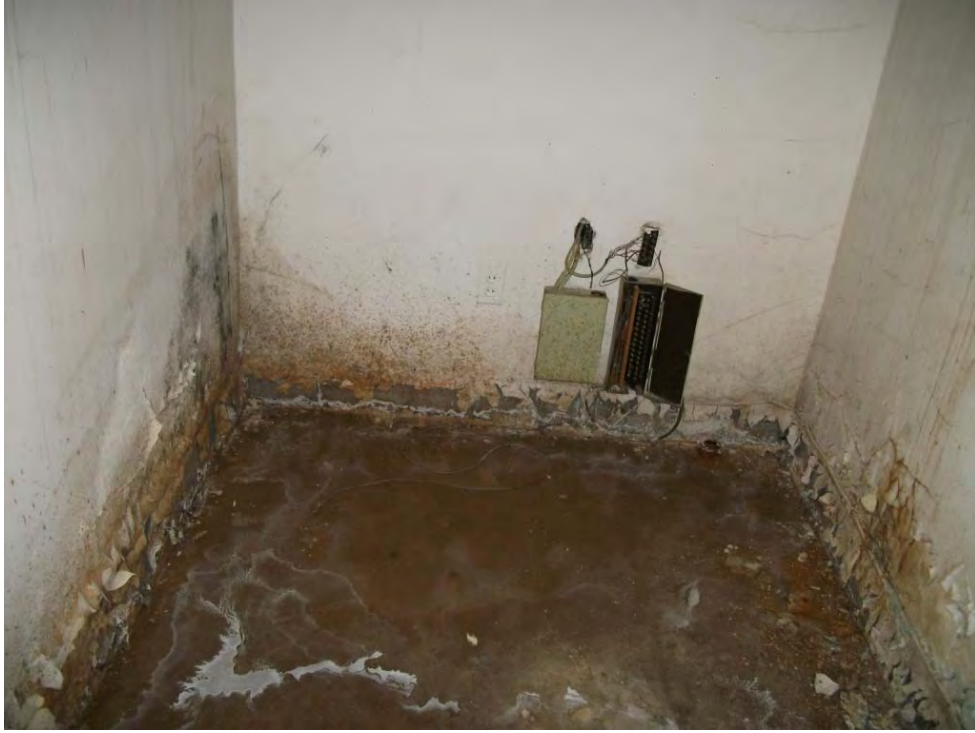
Basement East End Room 004
