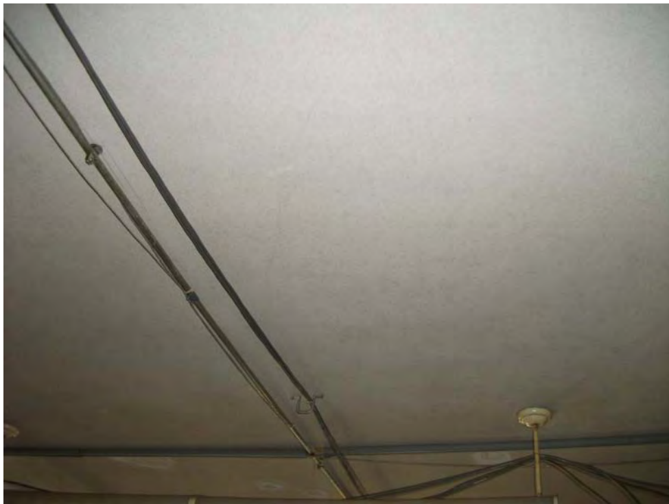
Basement East Side North End Ceiling
