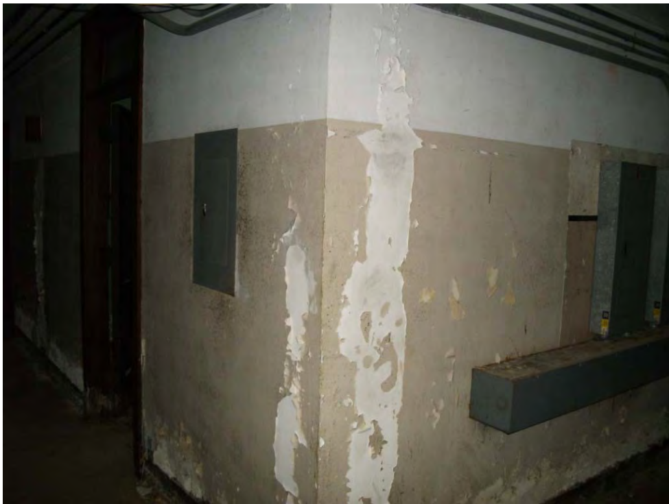
Basement West Side Hall
