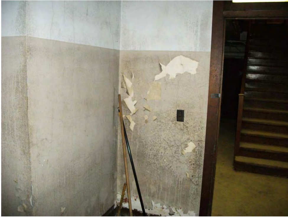
Basement West End Room 009
