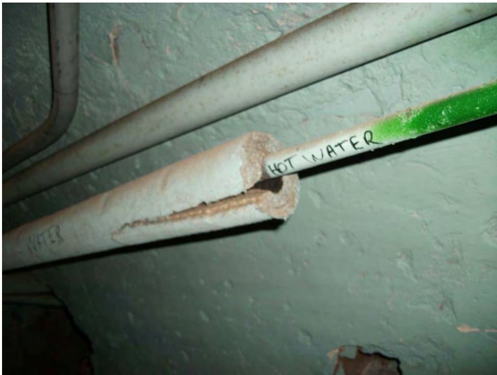
Homogenous Area J – Wrapped Paper Pipe Cover
