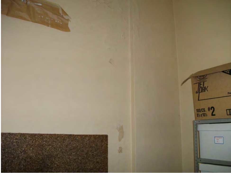
First Floor East End Room 134
