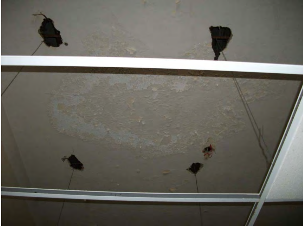
Second Floor East End Room 251
