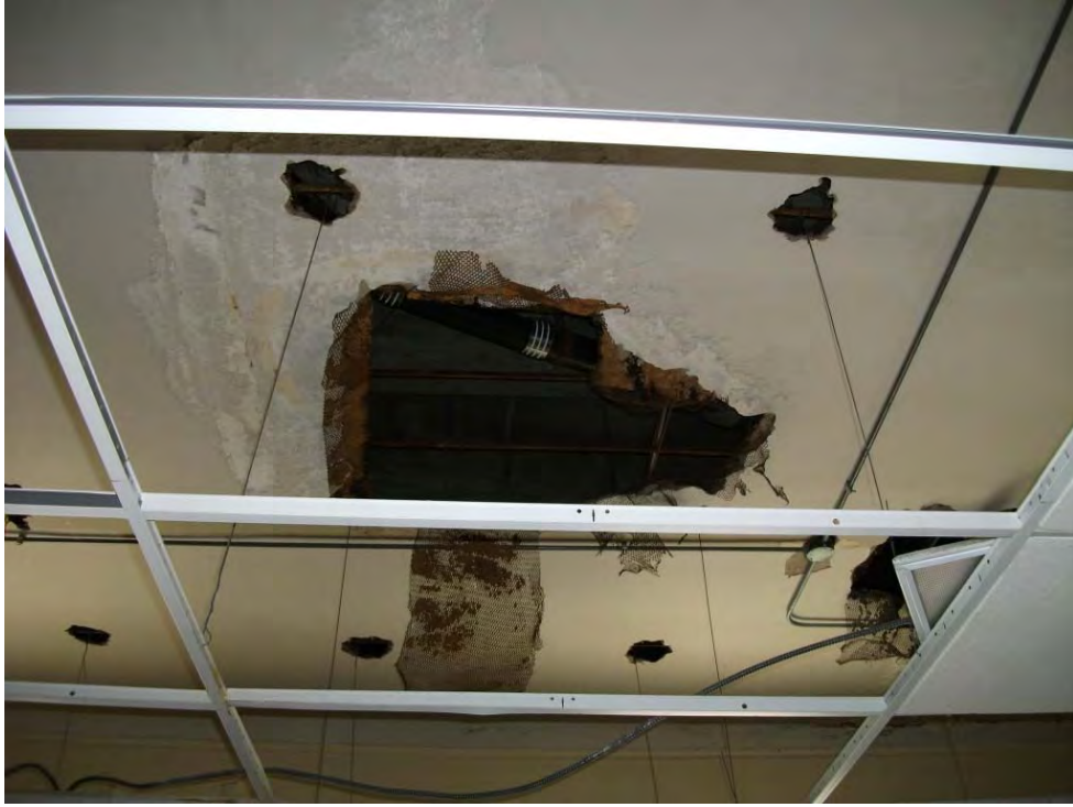
Second Floor East End Room 252
