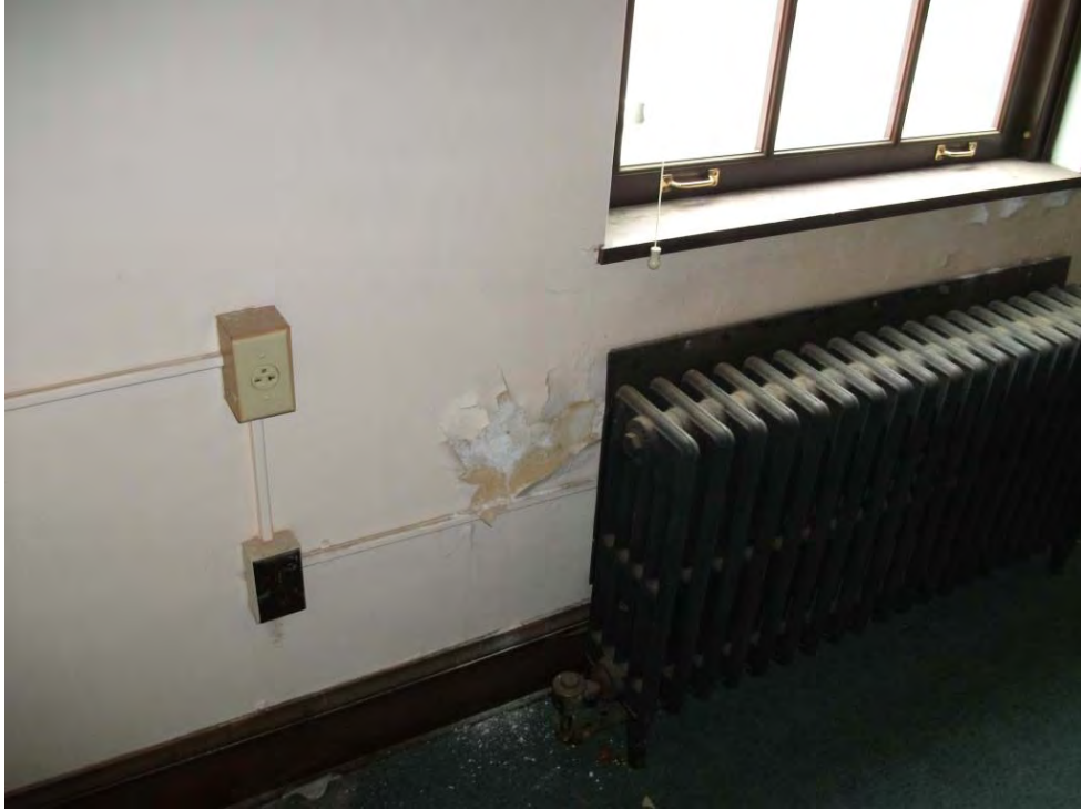
Second Floor West End Room 225
