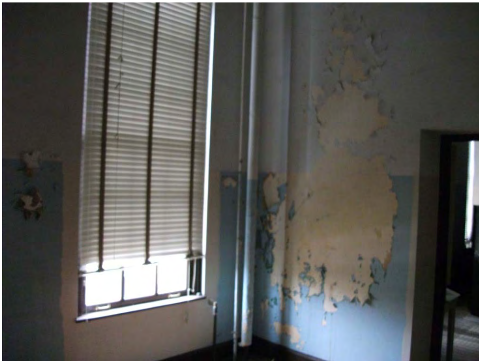
First Floor East End Room 130
