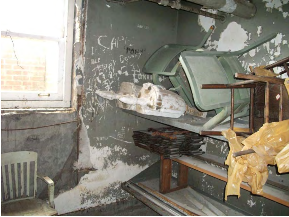
Basement West End Room 020
