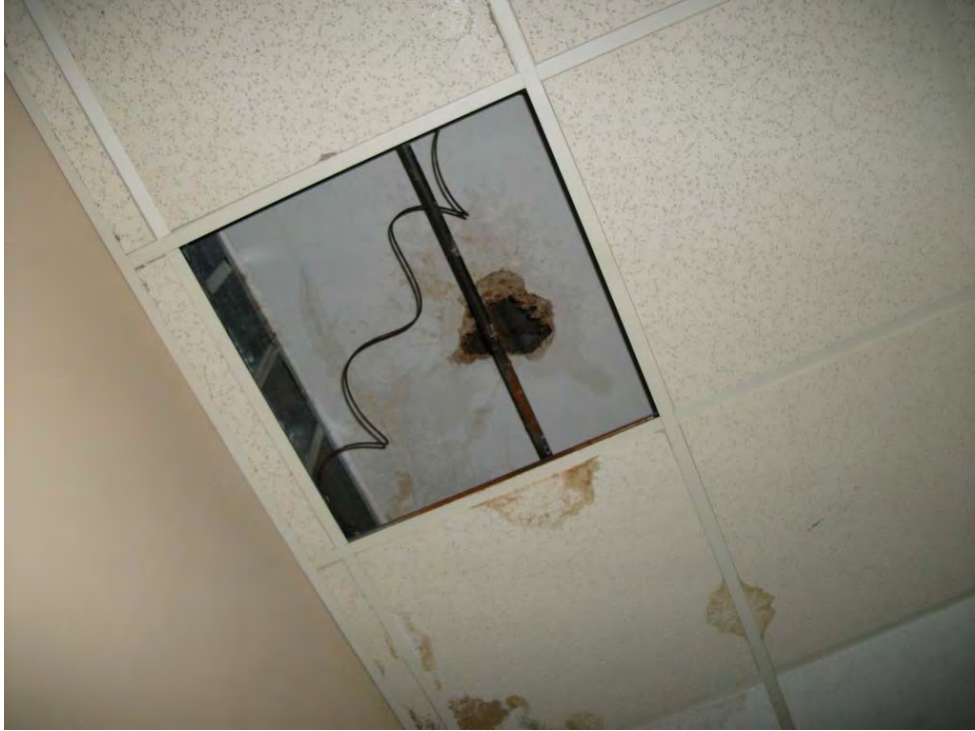
First Floor West End Room 115
