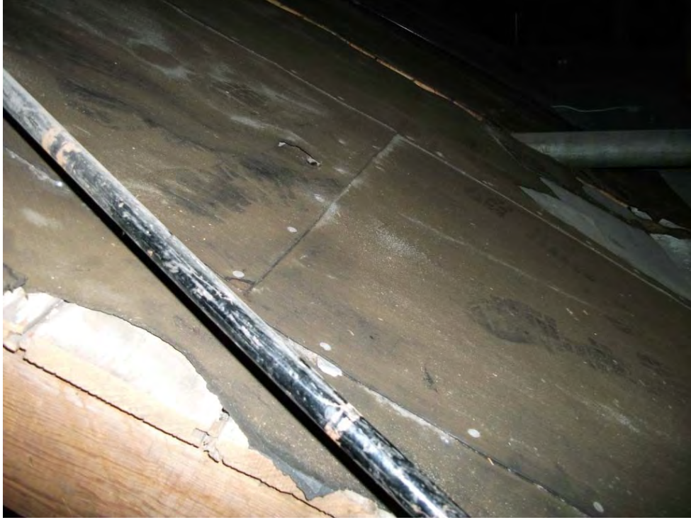
Homogenous Area Y – Roofing
