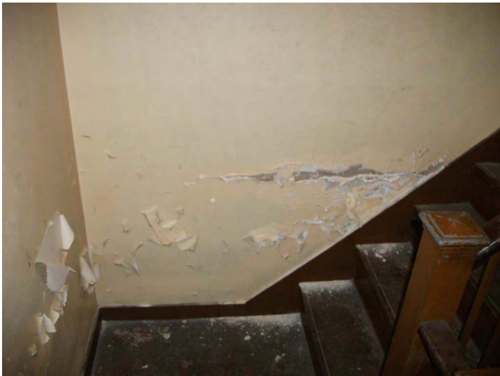
Attic Stairs East End
