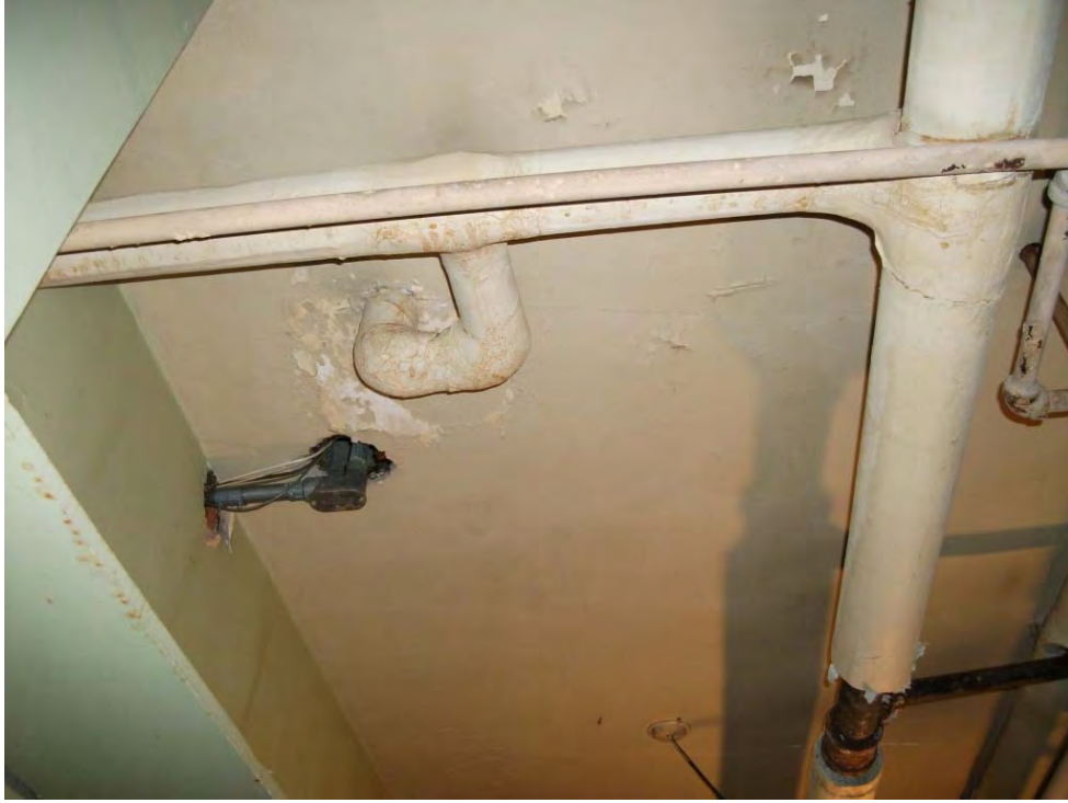
Basement East End Room 005
