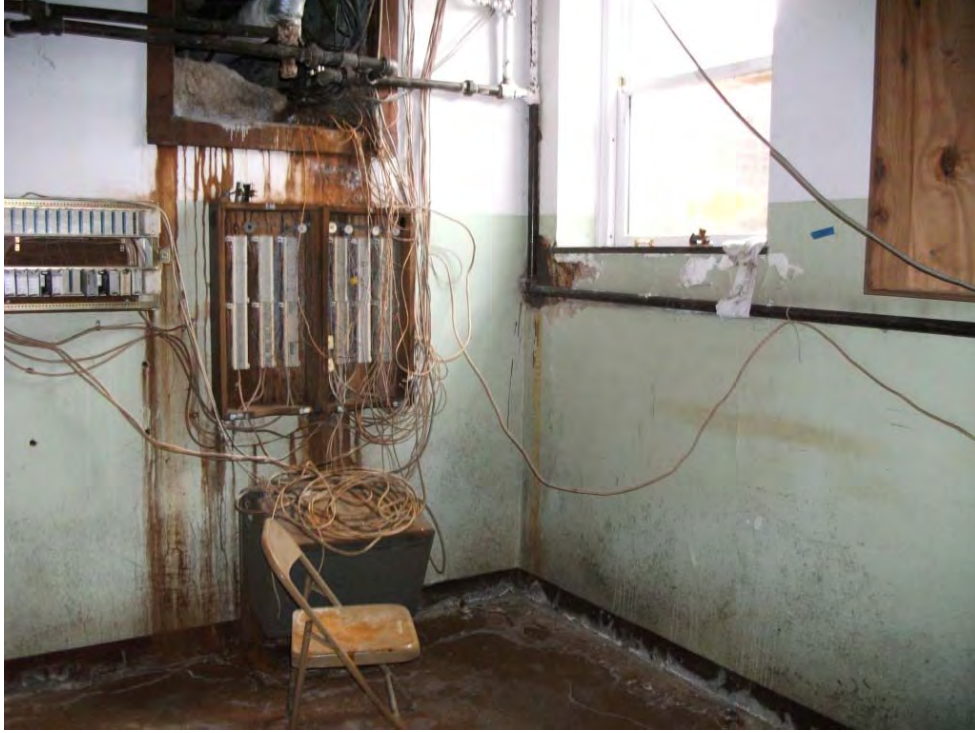
Basement East Side North End West Section
