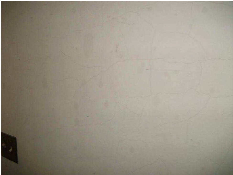
First Floor East End Room 108
