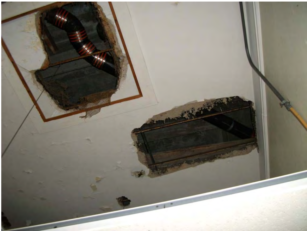
Second Floor West End Room 225
