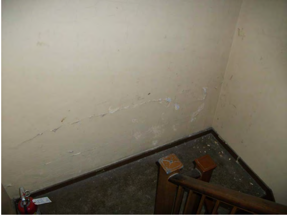
Attic Stairs West End
