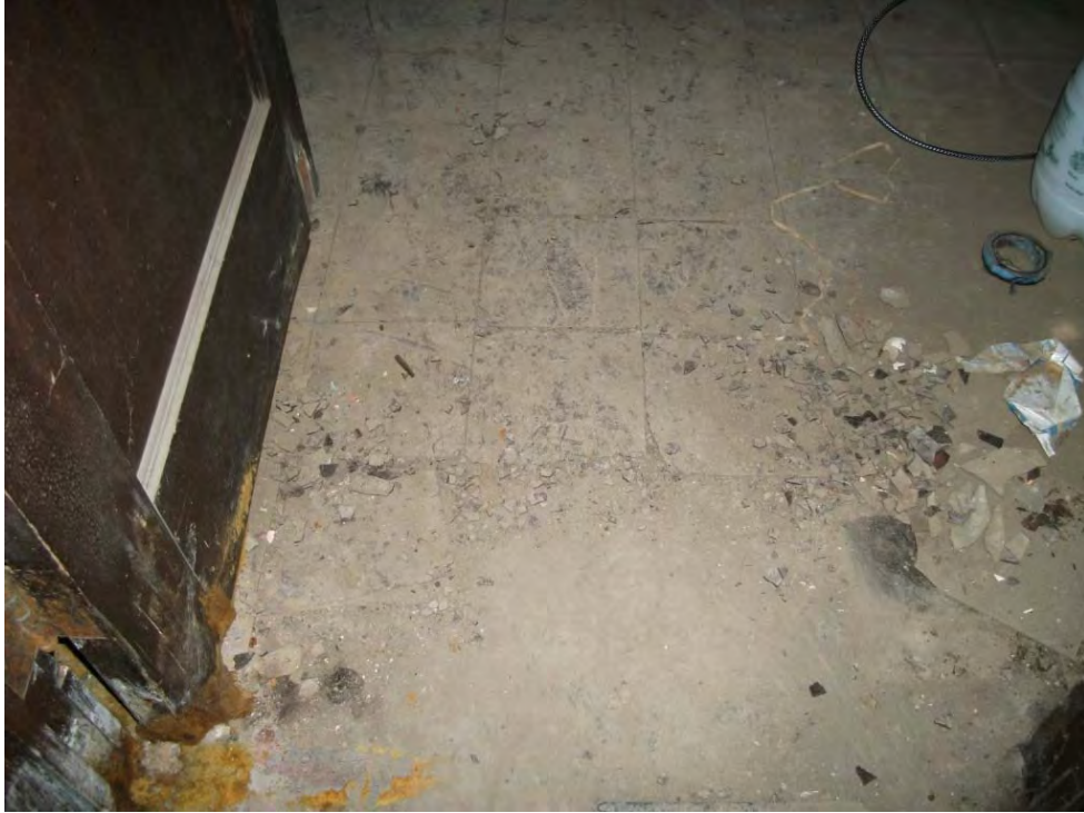
Homogenous Area A – 9x9 Vinyl Floor Tile
