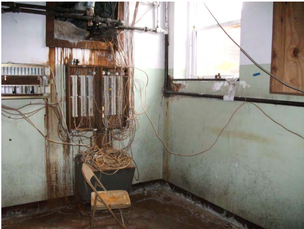
Basement East End Room 003
