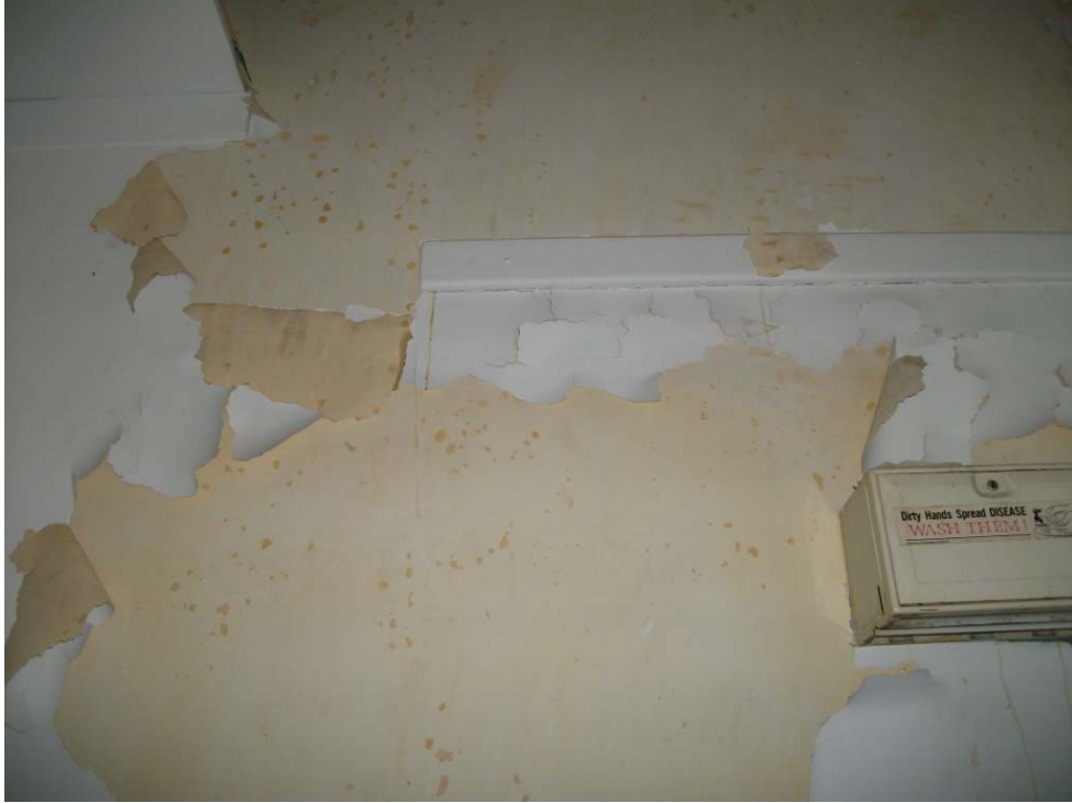
Second Floor East End Room 242
