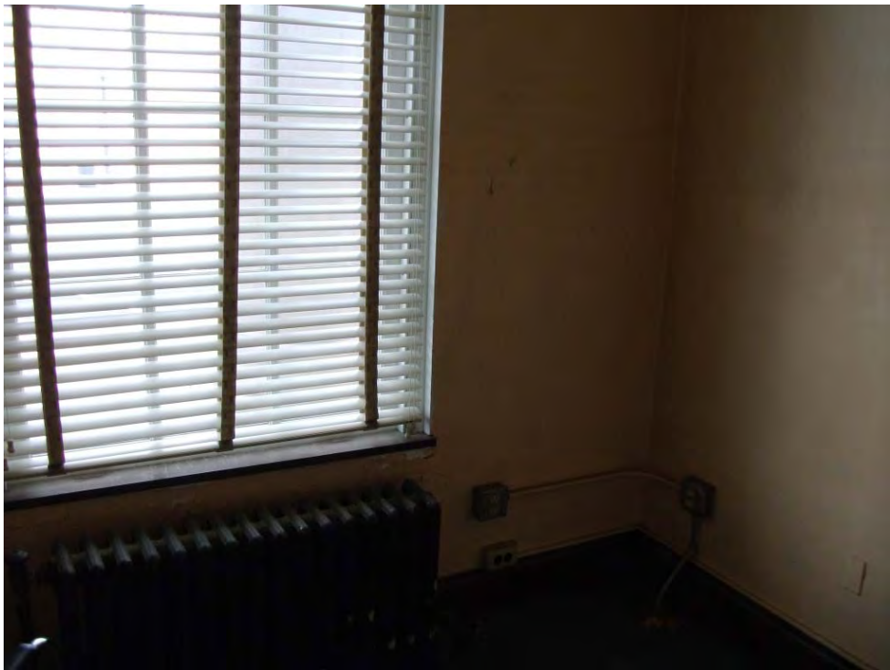
First Floor West End Room 144
