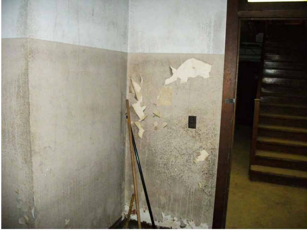
Basement West Side Near Boiler Room
