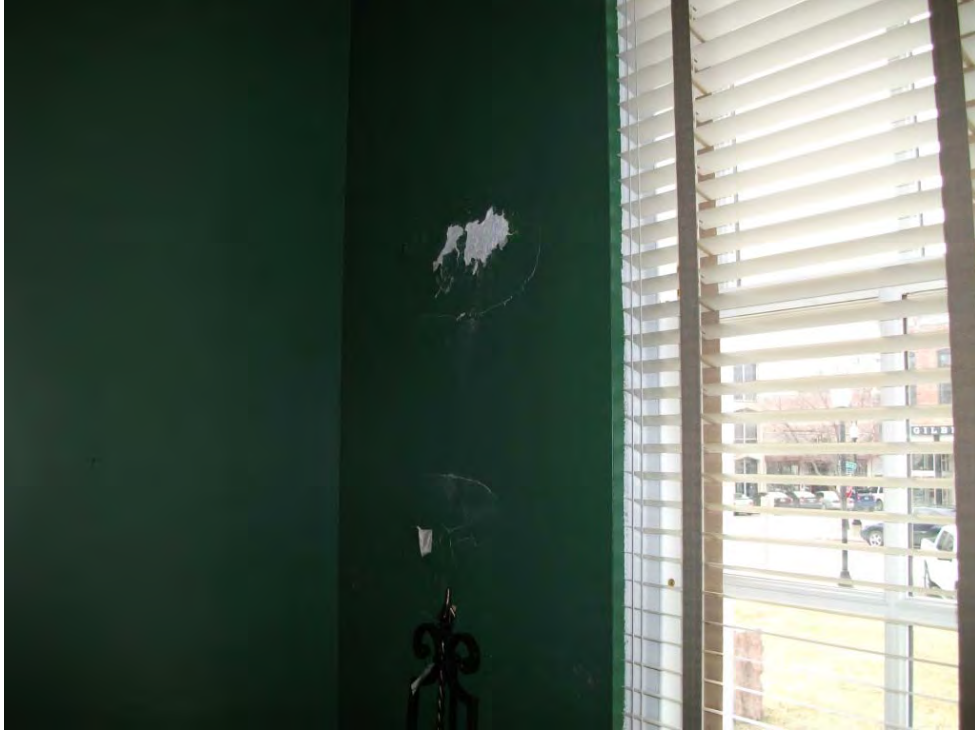
First Floor East End Room 114
