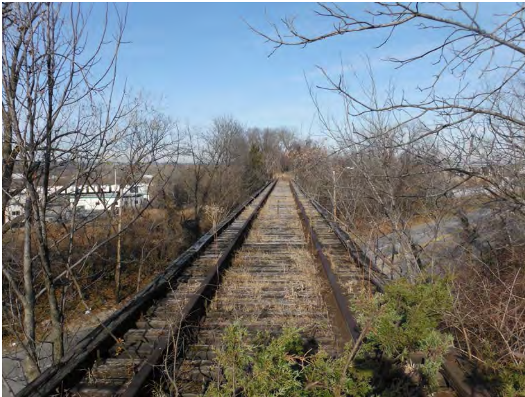
Photo 2: Rail bridge over East Stadium Drive, facing northwest.
