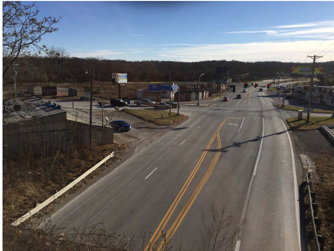
View from the deck plate girder bridge at Noland Rd. and 350 Highway, looking northeast.
