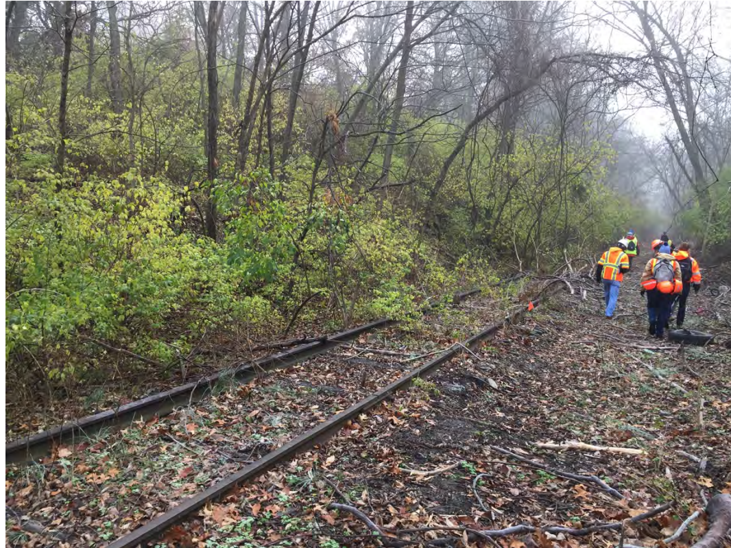
View near Larson Ave., south of East 75 th St.; looking southeast.
