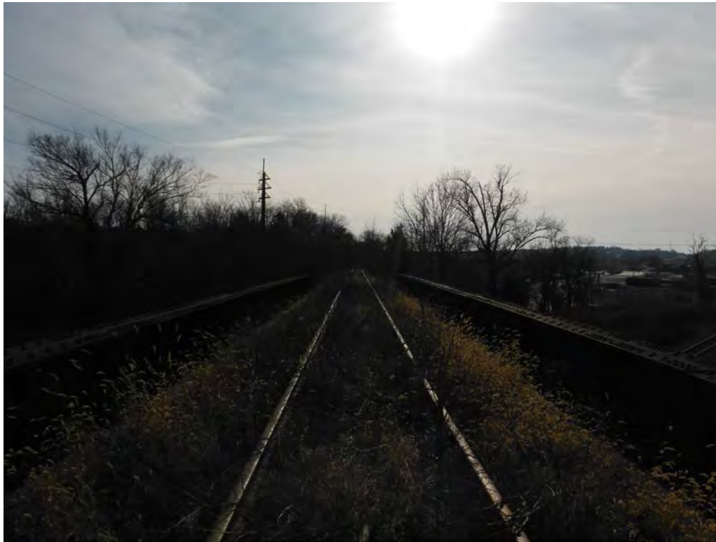
Photo 1: Rail bridge over East Stadium Drive, facing southeast.
