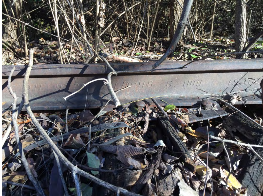
Detail of rail branding for 1930 rail; near Raytown Rd. and East 57 th St.
