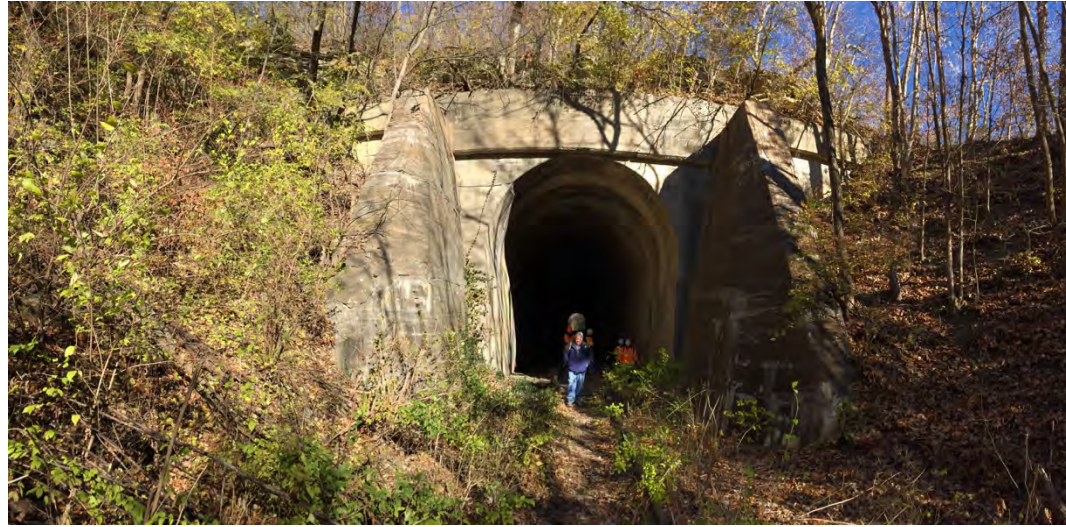
Panoramic view of Vale Tunnel, looking north.
